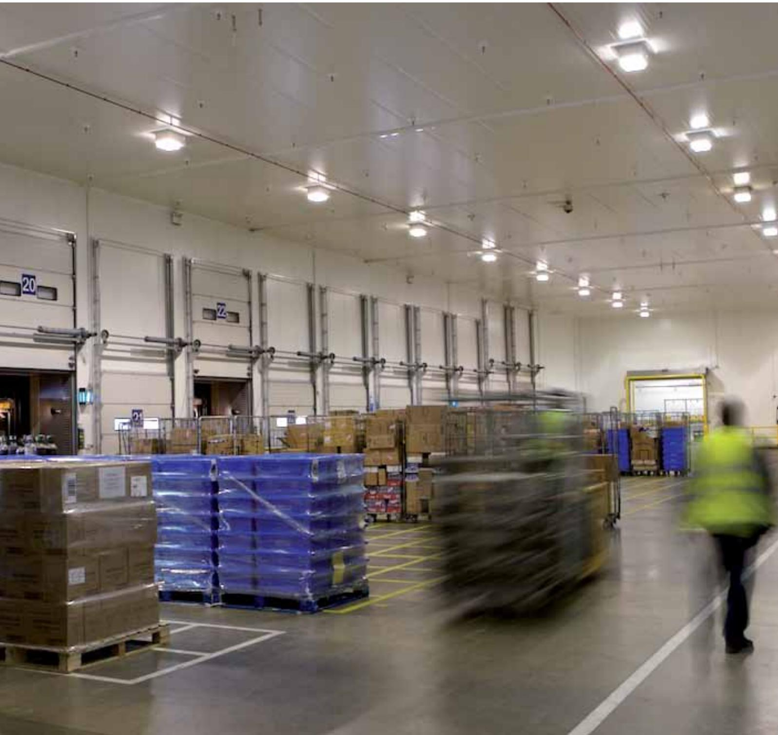
Lopak II is a robust low bay luminaire that is versatile for mounting heights over 5m, in a wide range of applications including factories, warehousing and retail
